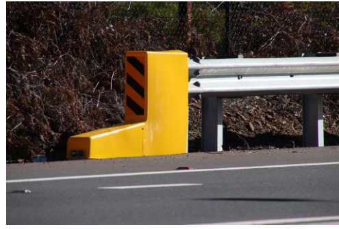
Guardrail End Terminal
